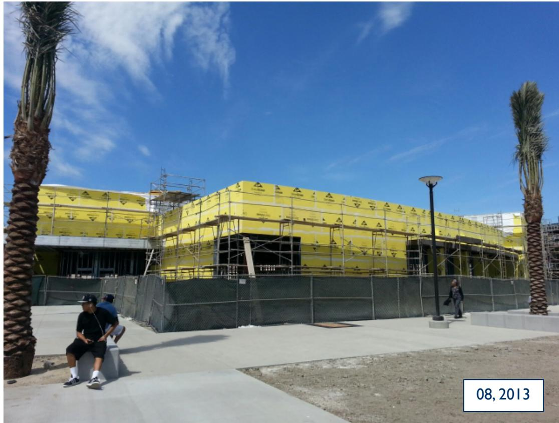
The steel stud framing and exterior gyp board installation is complete. The mechanical, electrical and plumbing rough-ins are proceeding.
