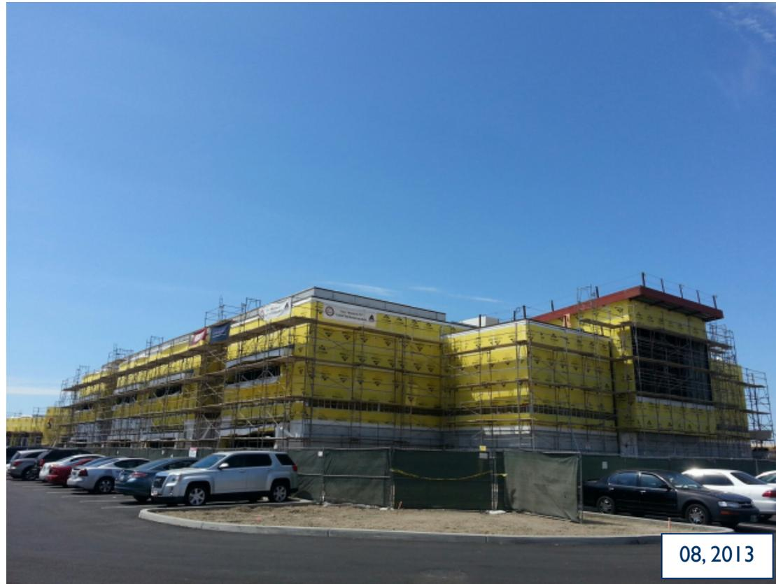
The Science Building has steel stud framing, exterior gyp board, and the mechanical, electrical and plumbing rough-ins completed. Insulation is installed and currently interior gypsum board is being installed.
