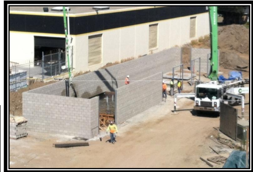
Foundations, CMU wall enclosure, and underground electrical vaults for the utility yard have been installed. The yard will enclose the relocated electrical gear and gas meter.
